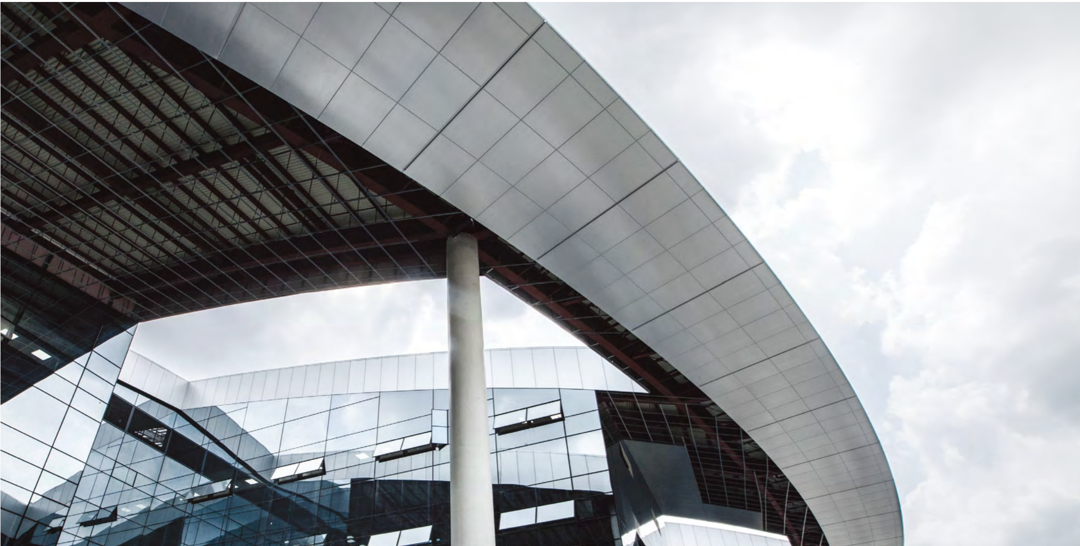
Exterior of Hankook Technodome
