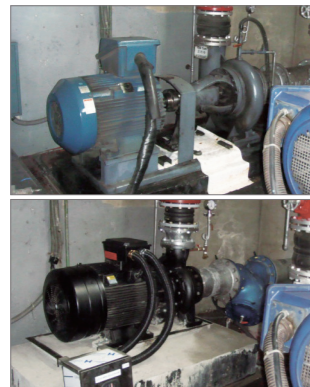
Before and after improving elevated water tank pump
